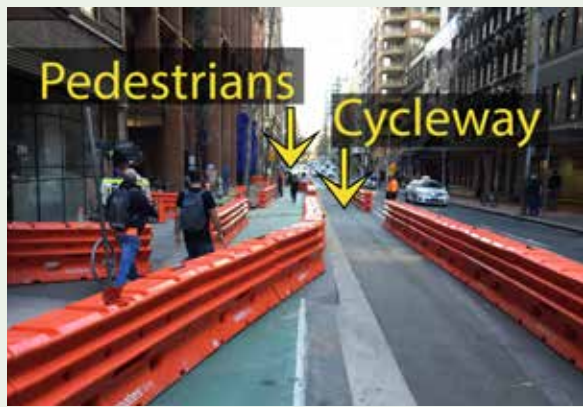
Figure 16(b): Temporary pedestrian and cyclists diversions should be avoided. Where works are proposed that require temporary closure of footways/cycleways , the City may agree to temporary diversions being established subject to meeting minimum design standards.
